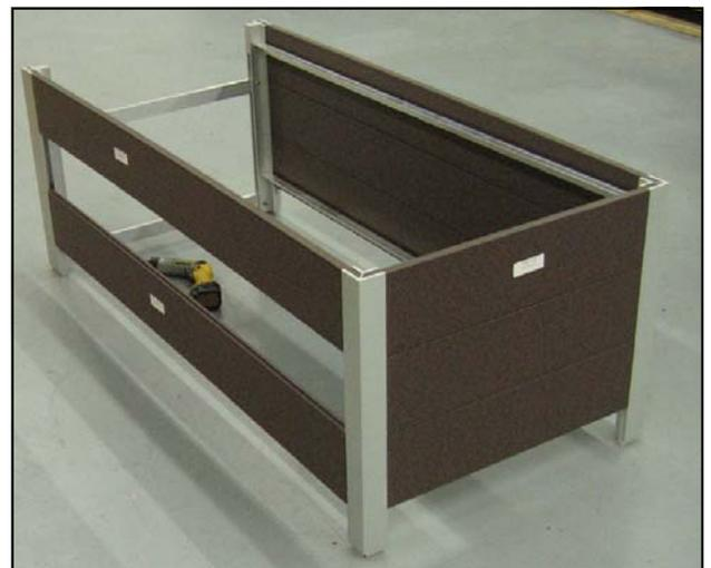
12) Gently insert the bottom back plank aligning the fastener holes, and lightly tighten with the screw gun on 3, then insert the top back plank leaving a gap between them. Next add the 3 at the front, again working from bottom to top. **Photos above right ^**
